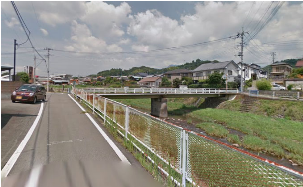
Fig. 1a The old Reiki bridge
