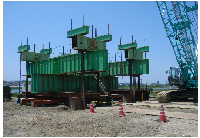
Figure 3. Photograph of the Static load test equipment
